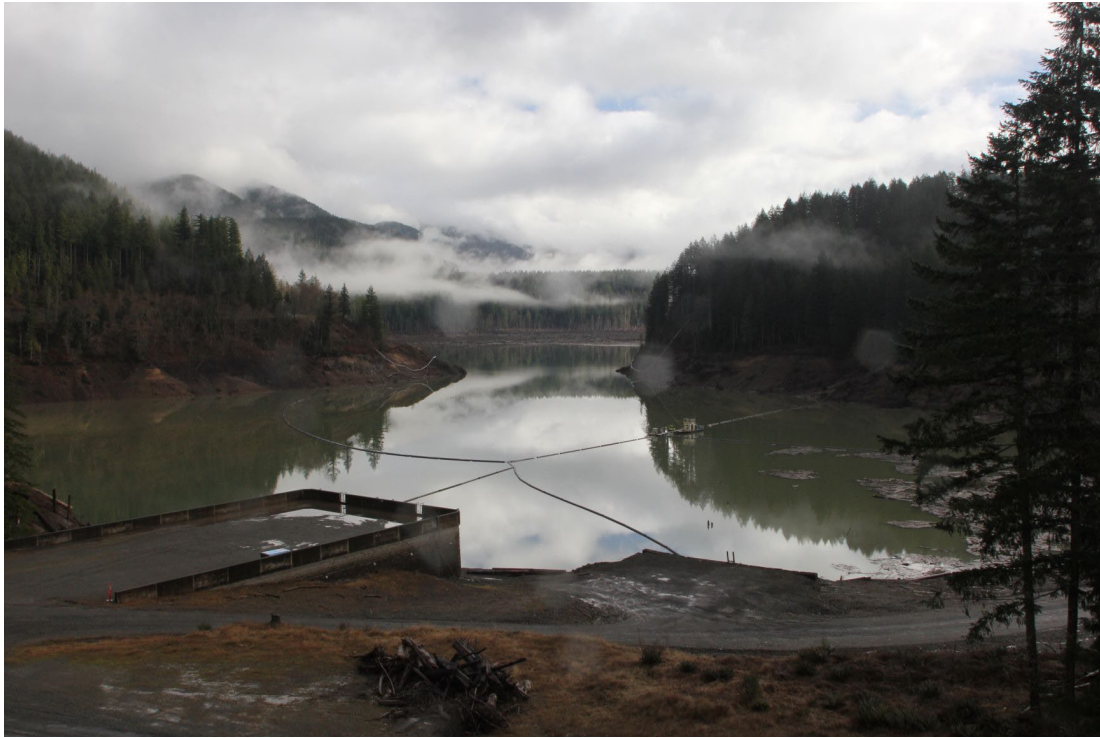
Figure 27. Boat dock area in January 2021. The lines visible in the reservoir are debris booms.
