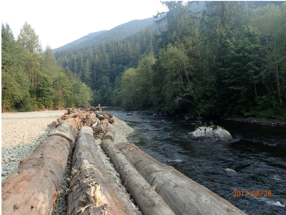
Figure 22. Large wood placed for downstream disbursement.
